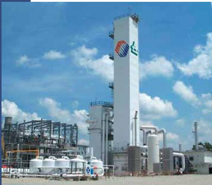
An Air Products/Cryolinfra nitrogen plant servicing the Jujo-Tecominoacan oil field in Mexico. The plant provides Pemex Exploration and Production pure nitrogen gas at a pressure of 4,300 psig for enhanced oil and gas recovery. The nitrogen injection process has benefited the customer by increasing their daily oil production more than 200% and natural gas production by more than 400%.
