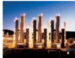
Located in western Wyoming, this nitrogen rejection unit processed up to 300 MMSCFD of EOR field gas for N<sub>2</sub> rejection and sales gas upgrading.
