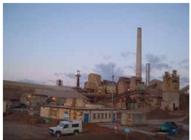
Figure 4. Steetley Dolomite's production increased about 10% with oxygen injection, restoring the performance they had before using alternative fuel.
