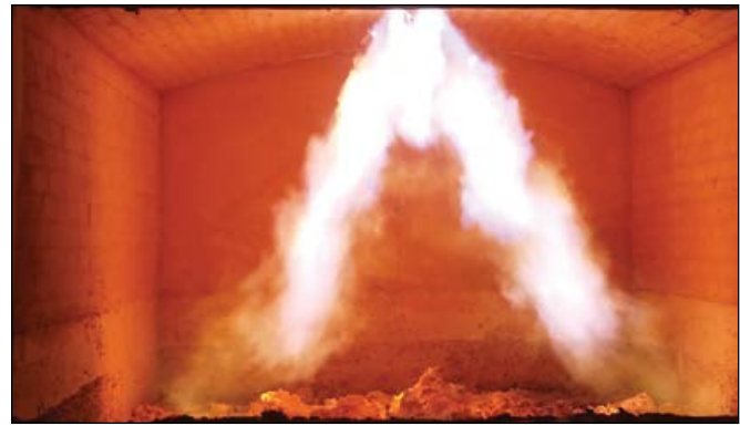
Figure 5. Photo of the Transient Heating burner operating in an aluminum reverb furnace.
